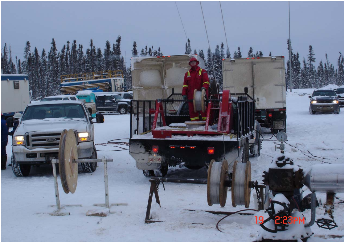
SHEAVES SET-UP ON SURFACE
