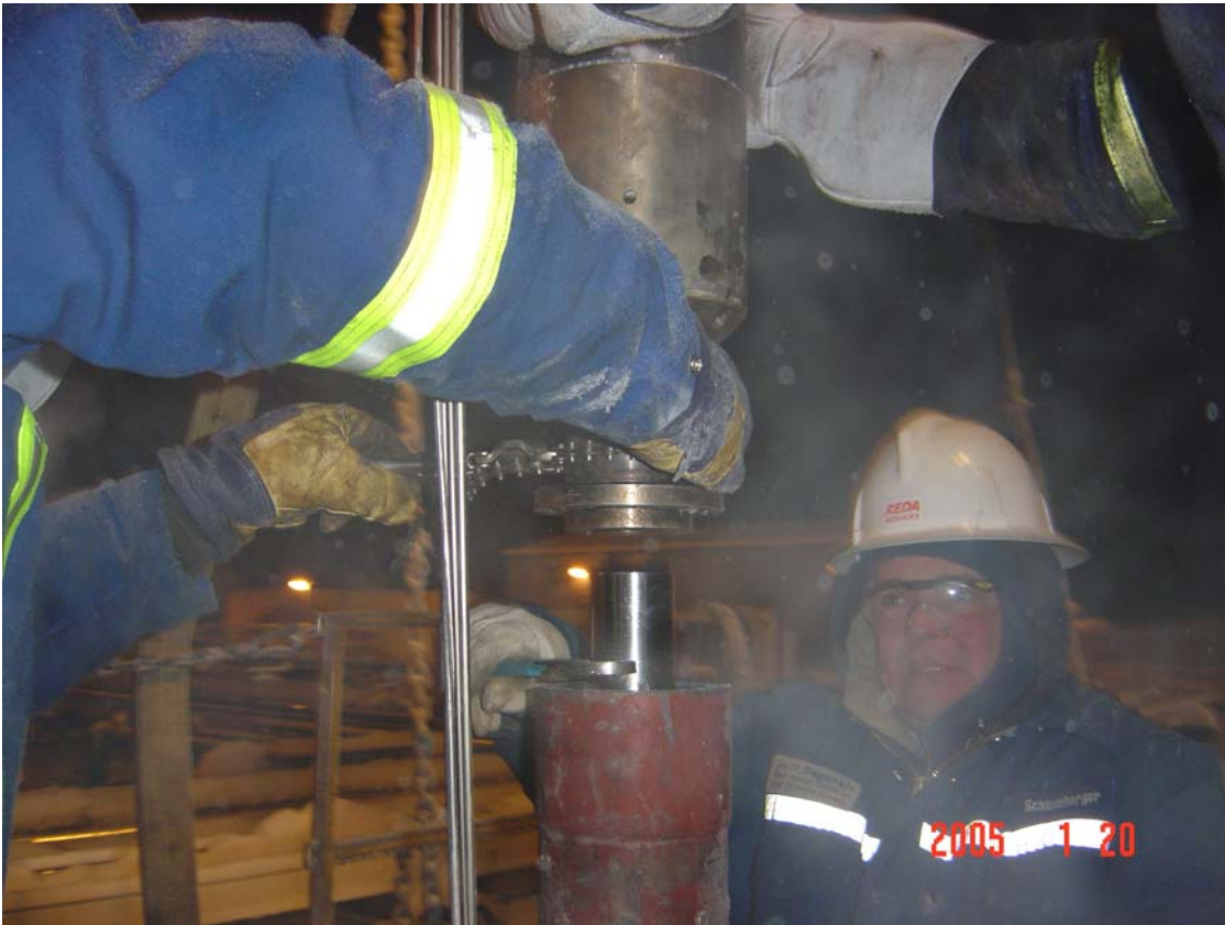
PUMP AND PROTECTOR BOLTING TOGETHER
